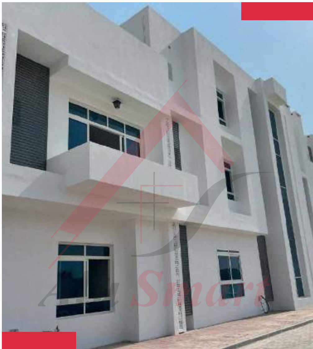
Project Name : Shiekh Salman Al-Thani Villa
