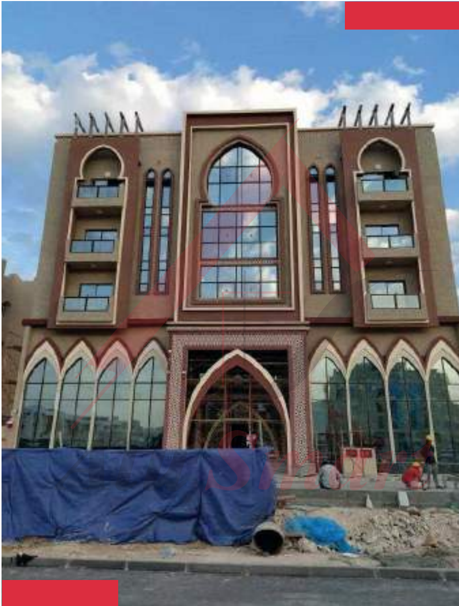
AlWakra Hotel . Main Contractor Sak Co
