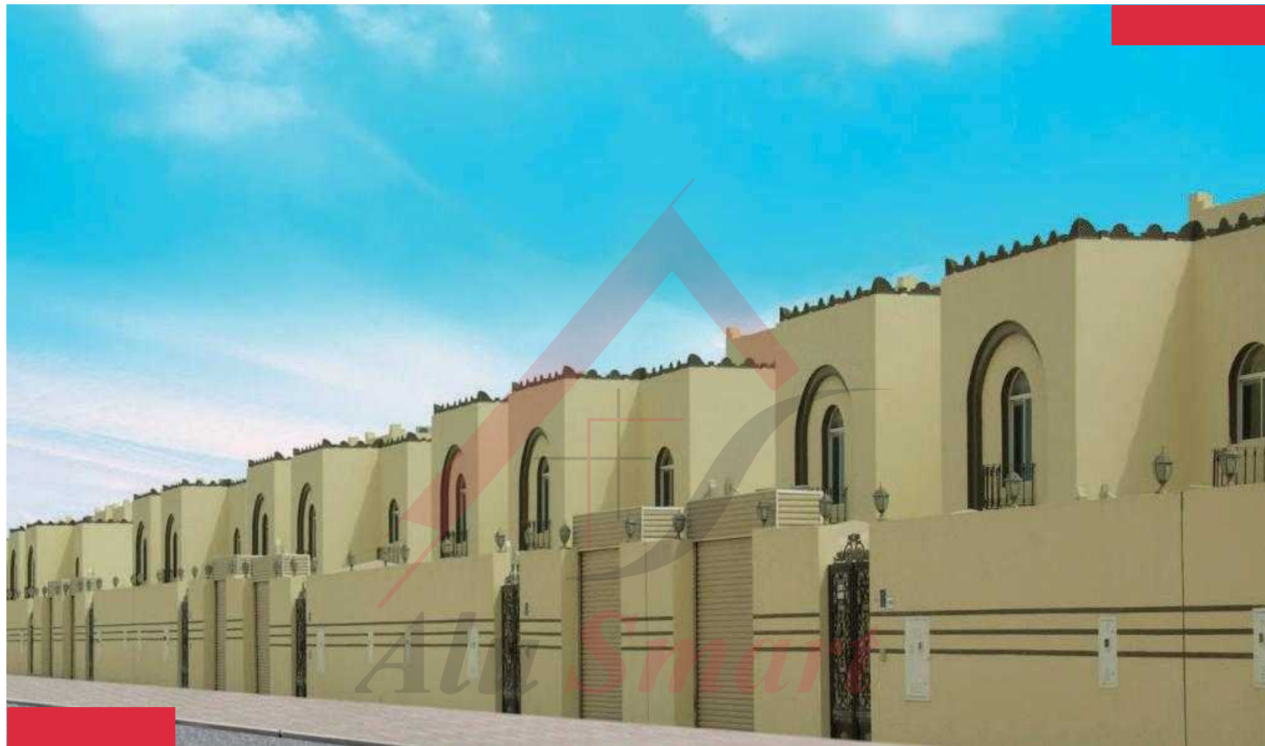
41 villas at Abo Salal mohamed ,Main Contractor ,Professional builder
