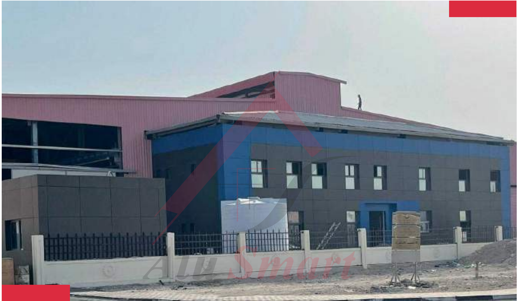
Negm steel Factory at New Industrial Area
