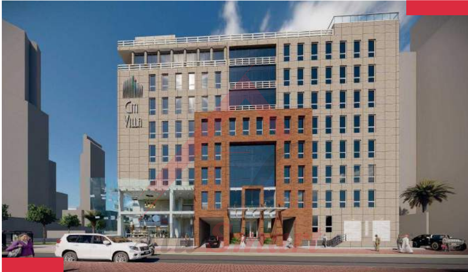
HAFSA Building Project ,
