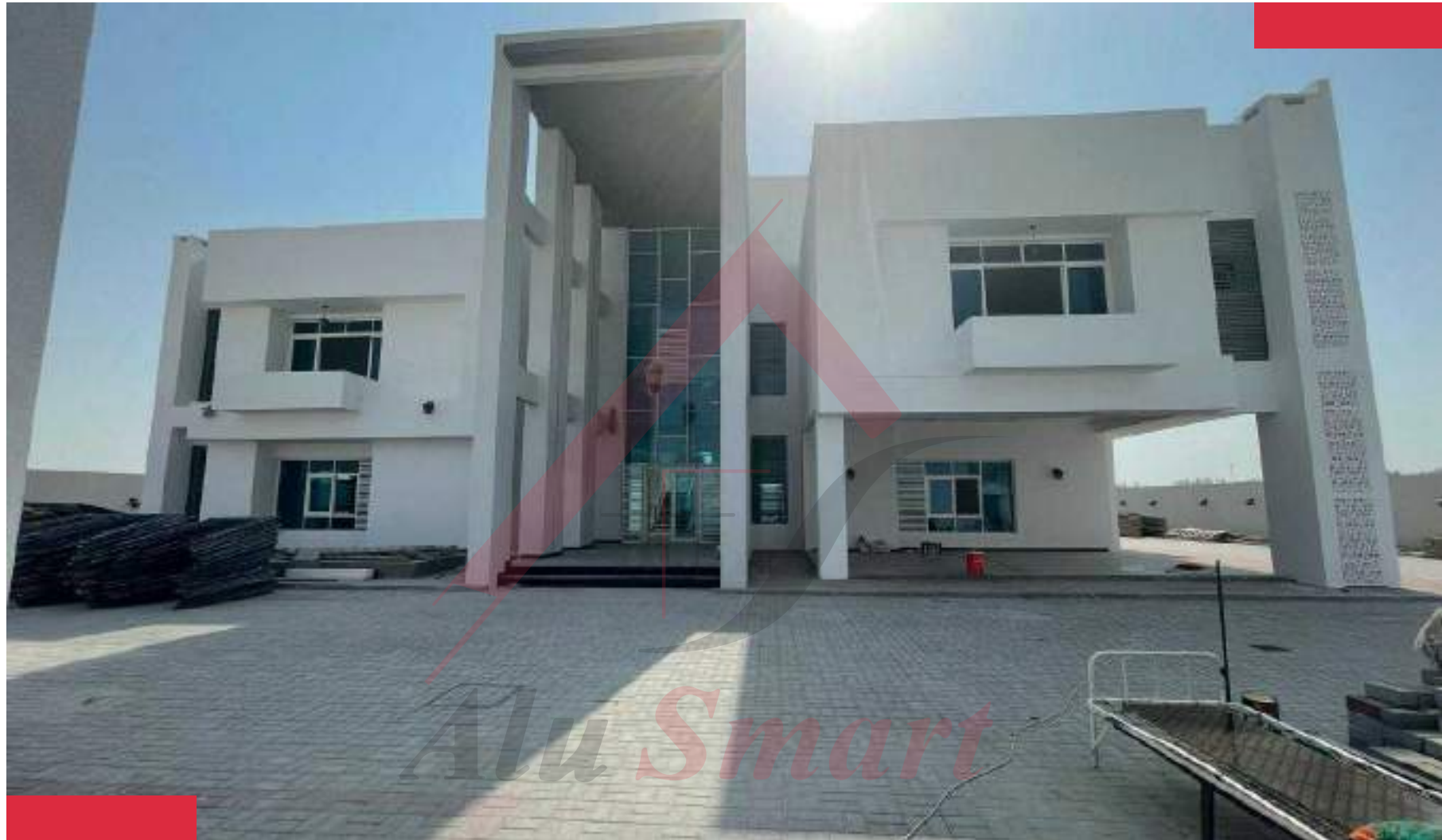
Project Name : Shiekh Salman Al-Thani Villa
